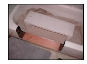
Tub Wall End Plug: cut a  $2 \times 6 \times 12^{\prime\prime}$  to fit into the tub wall for strength, and to anchor the end of the insert to with a screw and gray cap.
